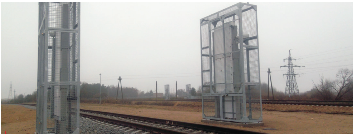
Special equipment records a violation, photographs the suspected vehicle or person, closes the road off with barriers and transmits all the relevant information to the central emergency warning station.
