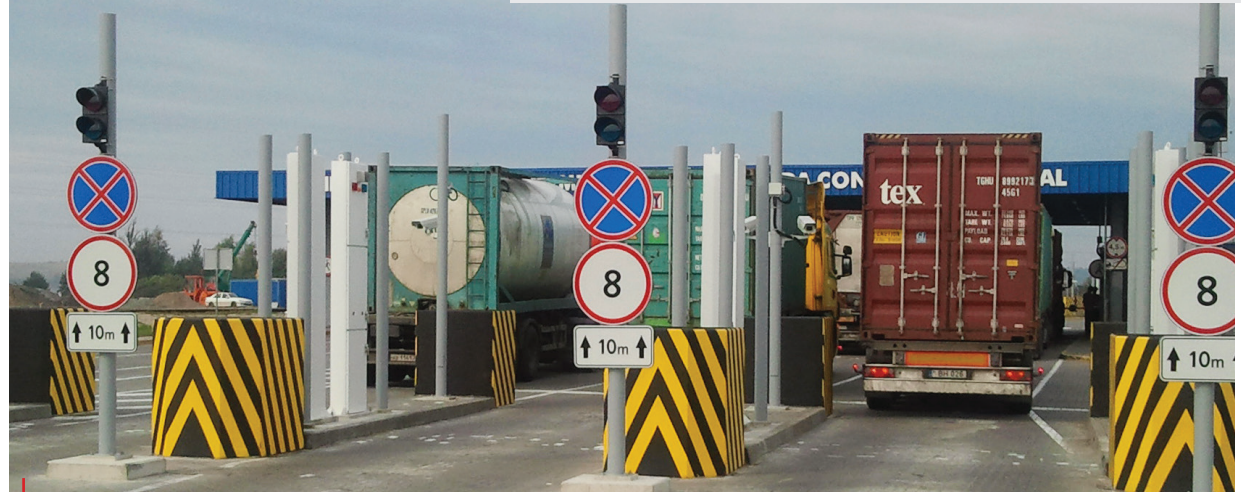
Different port areas now feature 25 radiation control gates comprised of three different types: for cars, pedestrians and trains.
