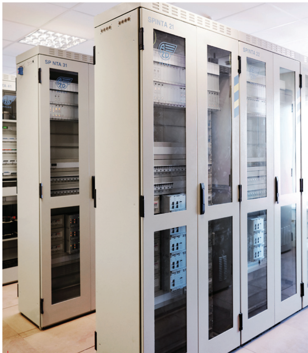
The modern microprocessor-based rail traffic control system has replaced the electrical and electromechanical systems that had been used for more than 30 years
